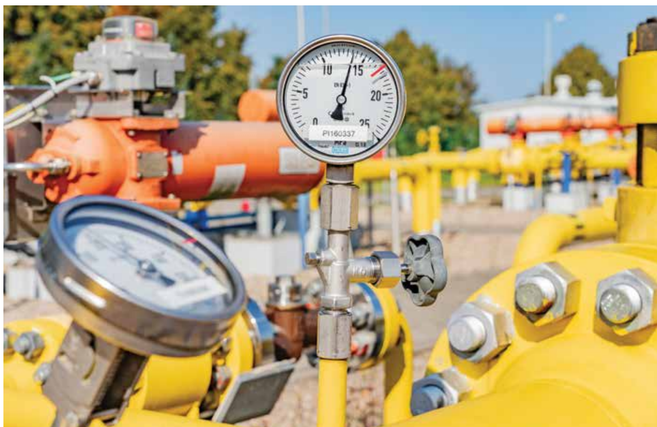
Fot. Gas Storage Poland sp. z o.o.
